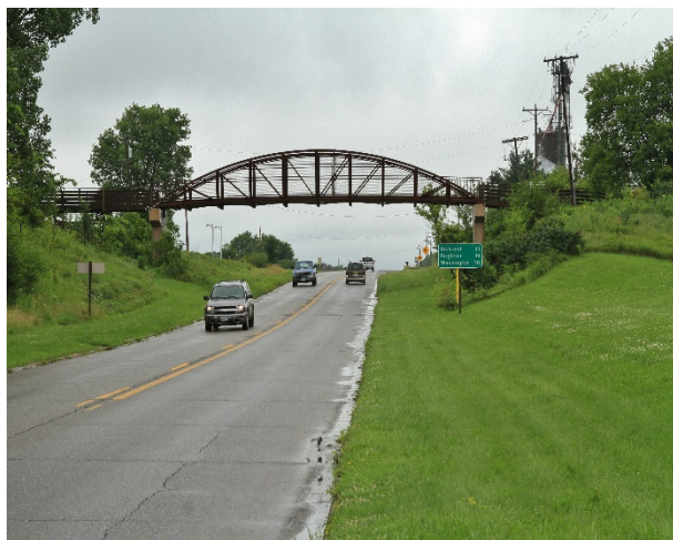
Matkin Bridge over Highway 1 north of Fairfield. This bridge project received $125,000 in Regional Enhancement funds from the RPA.
