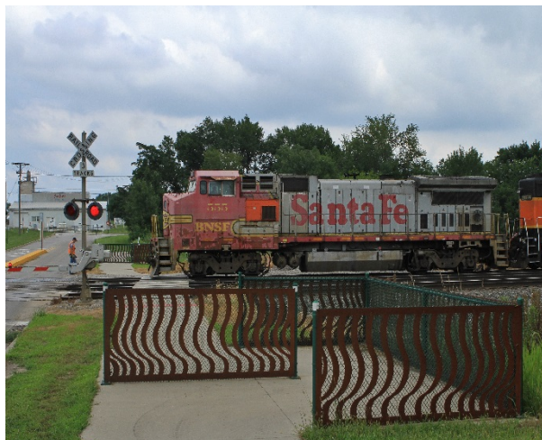
Railroad crossing maze safety enhancement along 28 th Street. Crossing maze incorporates Judy Bales Art.
